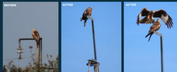
Fig. 5, 6 and 7 - Red kite released by the Eurokite LIFE project, with the wing tag X, in an electric pylon. On the left the electric pylon was before the correction by E-Distribución. On the middle and on the right the electric pylon was already been corrected and it was added a birds' perch, increasing the distance between the bird and the critical area of the pylon.
