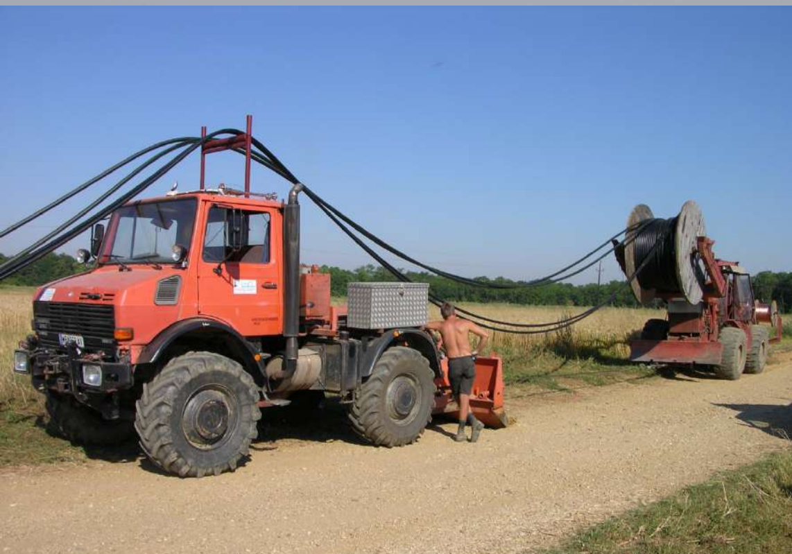
Underground cabling of a overhead power line in Burgenland 2006
