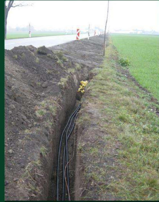
Underground cabling of power lines in Austria
