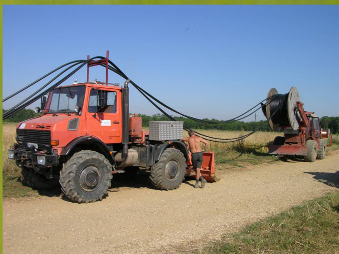
Transferring below the soil and the subsequent removal of a medium voltage power line as well as the marking of a high voltage powerline.
