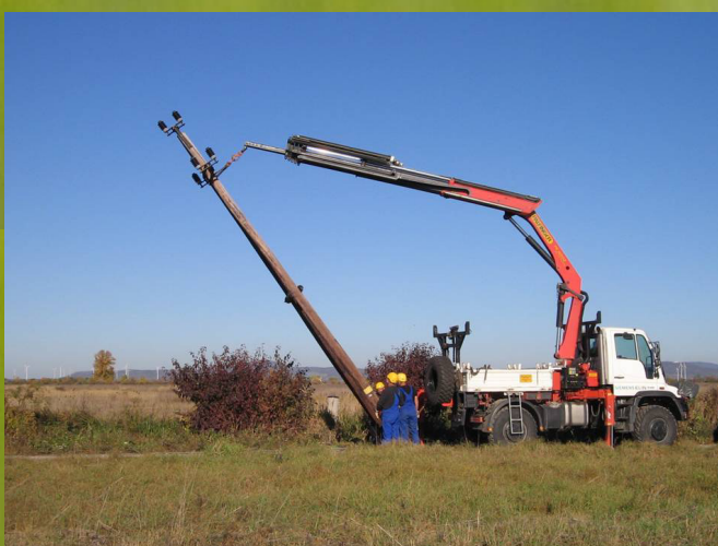
Transferring below the soil and the subsequent removal of a medium voltage power line as well as the marking of a high voltage powerline.
