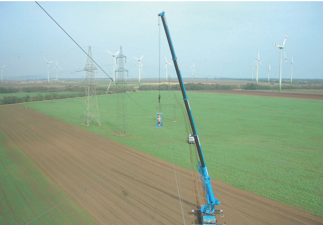
Marking of high voltage power lines with bird warning flags in the project area Parndorfer Platte-Heideboden in October 2007.
