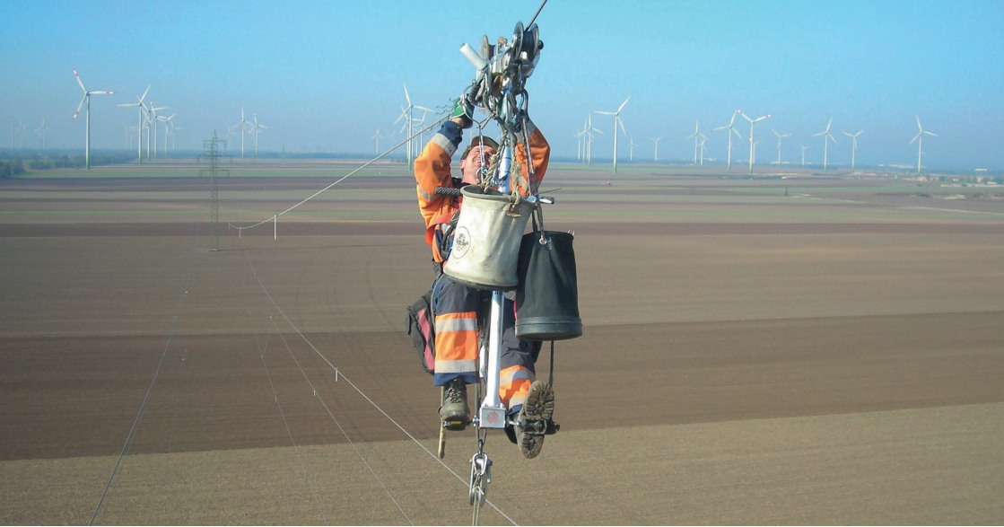
Marking of high voltage power lines with bird warning flags in the project area Parndorfer Platte-Heideboden in October 2007.
