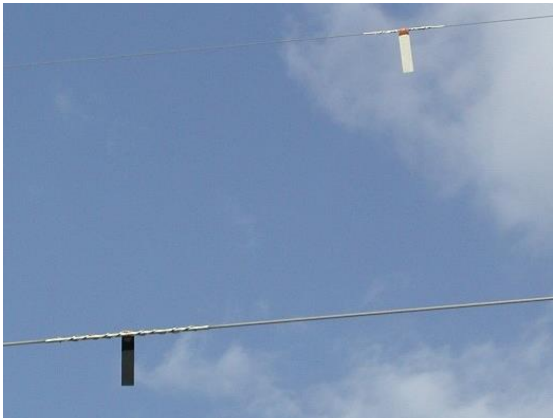
Figure 4: Bird protection flags on high voltage power line in Austria (Photo: H. Herzig).
