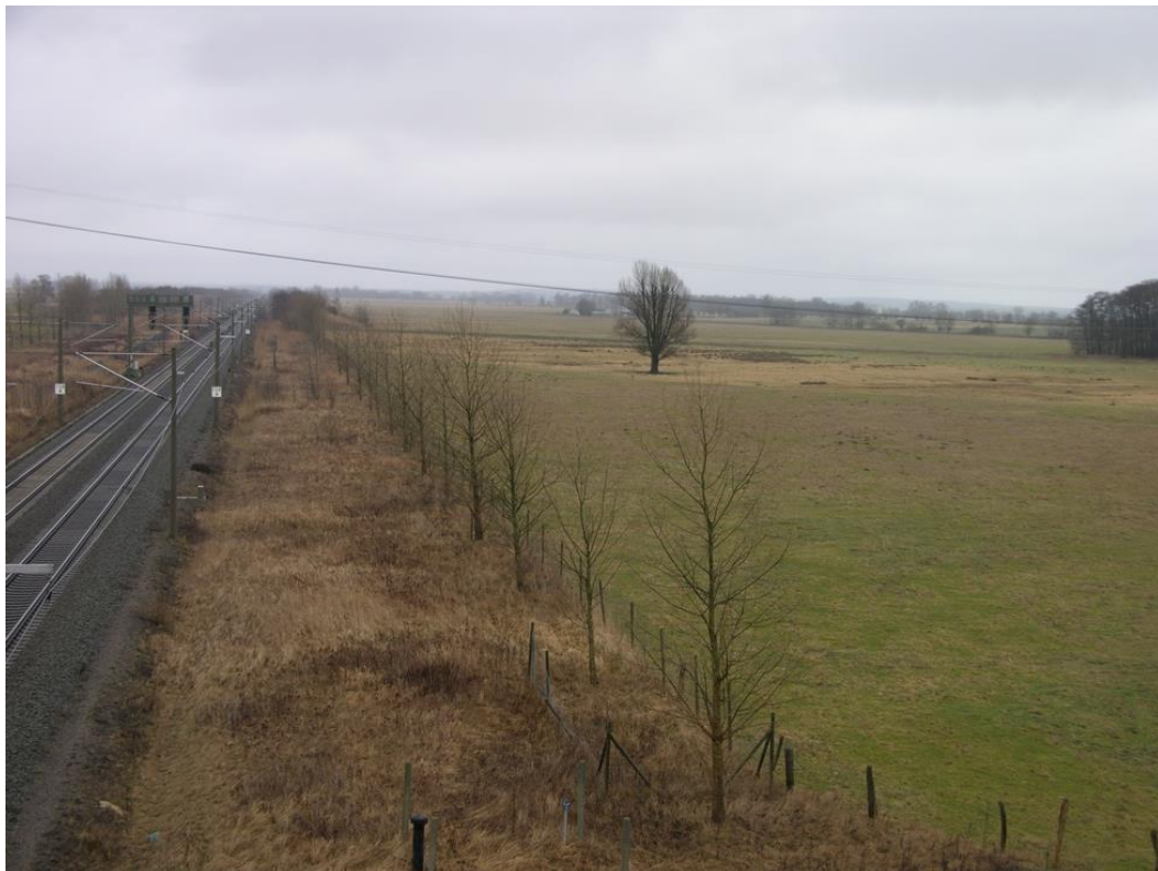
Figure 7: Planted shelterbelts in the Havelländisches Luch Great Bustard habitat, in Germany for „covering” the railway electric cables. Photo: Eike Julius.
