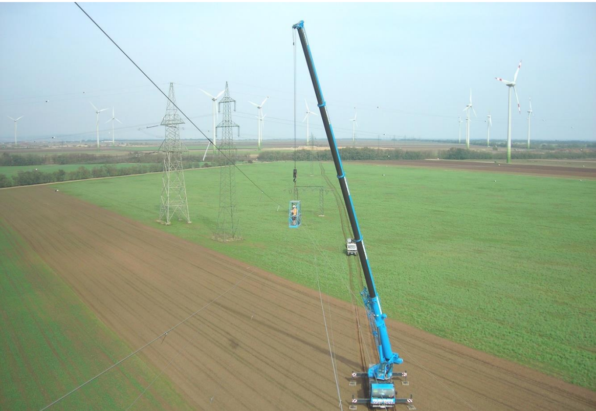
Marking of high voltage power lines with bird warning flags in the project area Parndorfer Platte-Heideboden.
